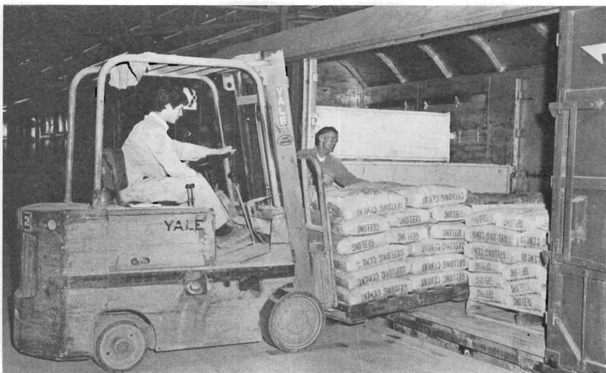
Palletized loading of bagged cement.
